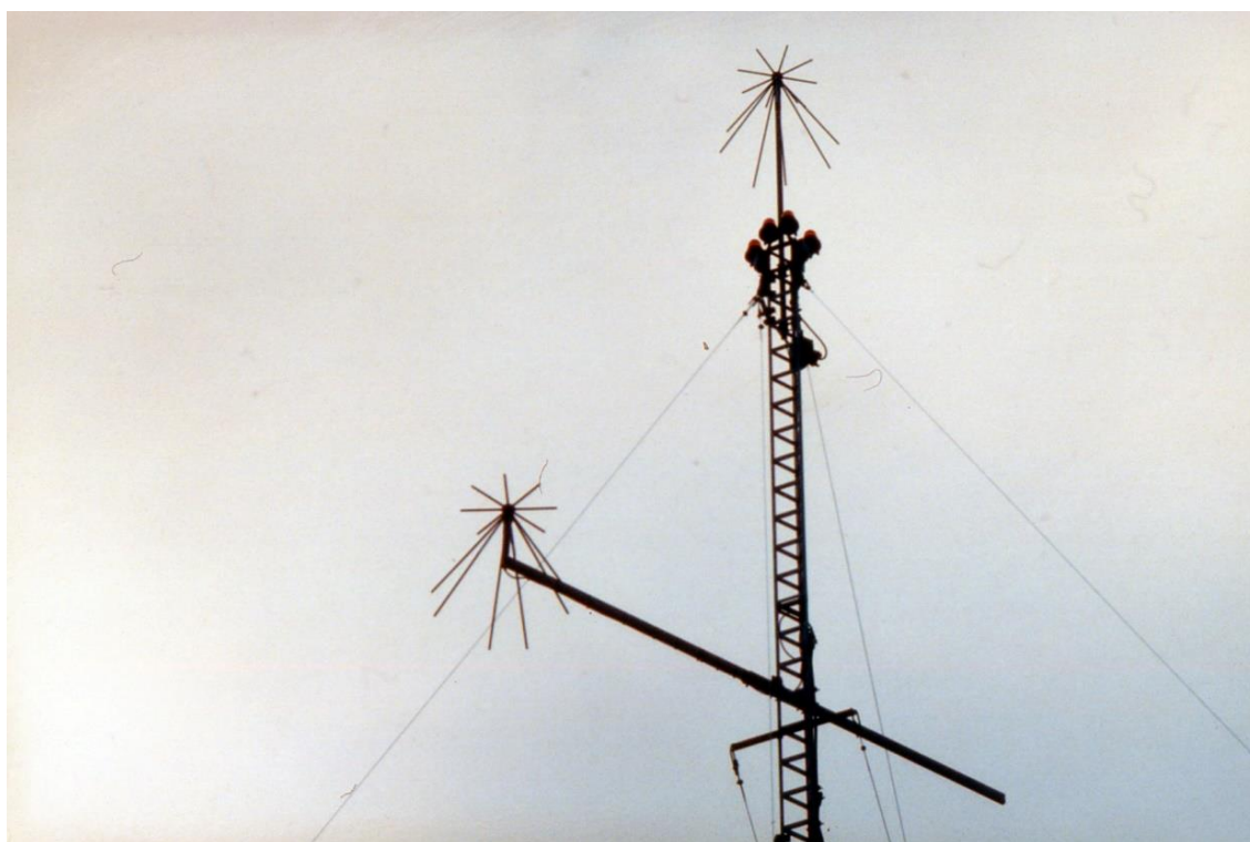
134. Kustradiostation mottagardel. UKV-antennor
