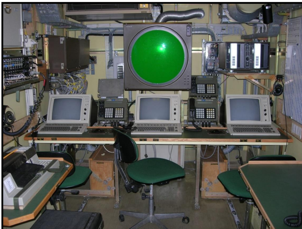
Installation i SLC-kärnan (Foto Malte Jönson)
